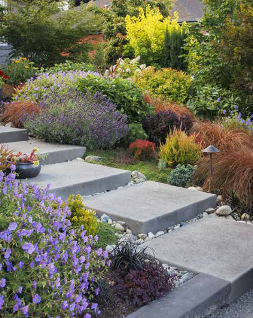
INNOVATIVE, MULTIFUNCTION HARDSCAPING ADDS INTEREST. Simplistic pavers could have been used to build the new front walkway, but poured concrete pads allowed the elevation change to be managed in a more beautiful fashion. Each landing is large enough for lingering, too, allowing visitors to take a closer look at the colorful beds on either side.
